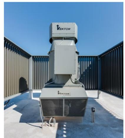
One of three Greenheck Vektor-HS fans installed to safely expel exhaust fumes from laboratories.
