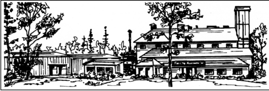
Main Office, Manufacturing and Warehouse Hanover, MA
